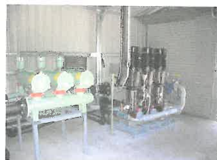
Byron Bay Golf Club installed a variable speed Rain Bird V-3300 pump which increased capacity to 30l/s
