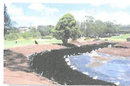
Construction of the lined irrigation pond which stores treated effluent
